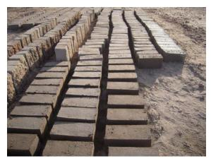
All blocks are made on site. It is the normal practice for contractors and that can mean the need for even more water to be available on site. The blocks are made in advance as they will take three days before they can be used.
