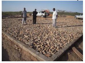
So our foundation is in and we are ready for the slab. Meetings on the site were regular between myself, the contractor, the engineer and the foreman. There are always details to be solved. When putting in the slab it is important also to mix an anti-termite chemical with the concrete. Termites can eat up a very good building in one year.
