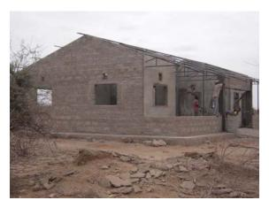
The roof is now in place and we are ready to put on the sheeting. The roof will be of corrugated iron but has the ability to reflect the sun. So normally you would expect a corrugated iron roof to make a building very hot but this particular iron sheeting reflects the sun.
