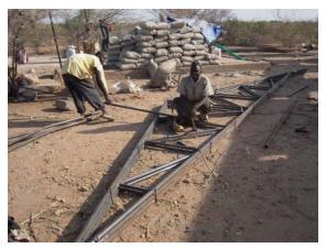
Because of the problem of termites we decided to make the roof with steel. It is an extra expense but in the long term it means termites cannot eat steel. The contractor brought his own welder on site which is another feat to be accomplished. A big generator and welding machine have to transport through the desert and across the dry river beds.
