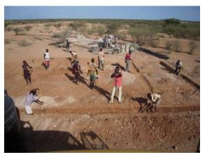
Blocks to be made and the site to be marked out in the early days. The actual site was very hard which is very good for the building but for the workers it was a tough task to dig out the foundations. No machinery on this site so the work is tedious in extreme hot
